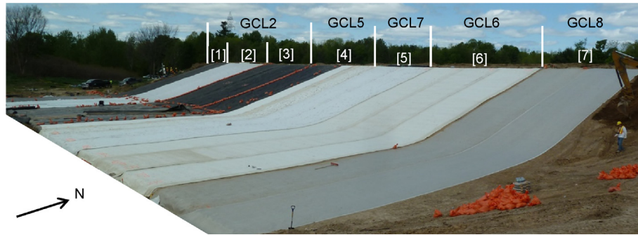
Fig. 15. QUELTS II during construction in May 2012. Textured 1.5 mm HDPE geomembrane was placed on the slope and a smooth geomembrane on the base. Sections from west to east (left to right): [1] GCL2 with 0.3 m gravel, [2] GCL2 with white GMB, [3] GCL2 (control; as per Section 3 of QUELTS I), [4] GCL5, [5] GCL7, [6] GCL6, and [7] GCL8 with polypropylene coating-up (Table 1).
