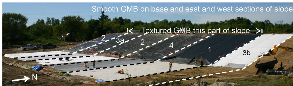
Fig. 2. QUELTS I during construction showing GCL and geomembrane layout. Each section had 3 panels of GCL. Sections (west to east): GCL2, GCL3a, GCL2, GCL4, GCL1 and GCL3b. The total lined width was 80 m.
