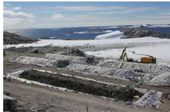
*Construction of the biopile. Filling biopile with excavated contaminated soil*
