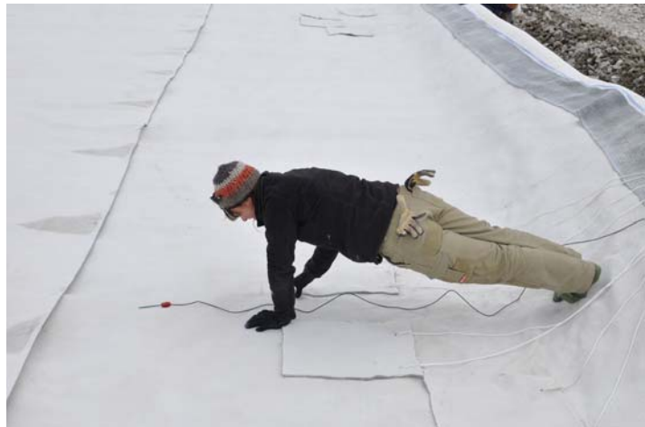
Rebecca installing sensors on the liner in Antarctica
