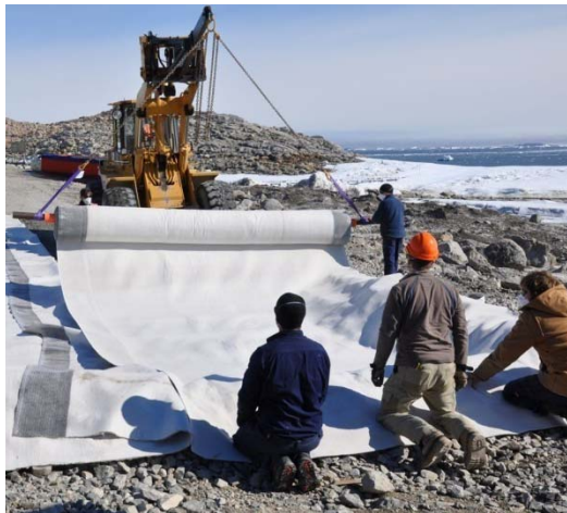
Liner construction in Antarctica
