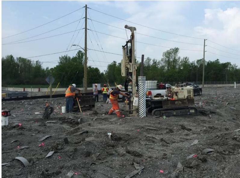
**Installation of vibrating wire piezometers with a Geoprobe geo-environmental drill rig**
