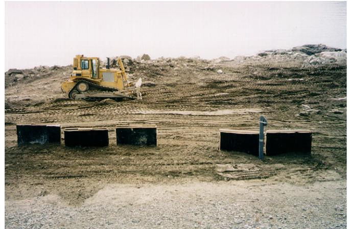
Fig. 1. Photograph of frames supporting f-HDPE GM coupons during installation and prior to complete soil burial and placement of GM surface cover.
